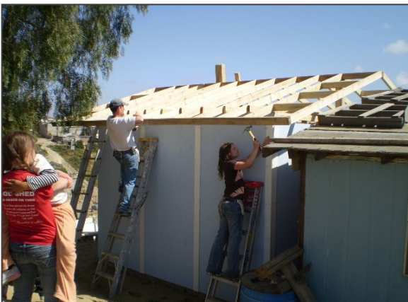
MOST Ministries Construction Team – Mexico
